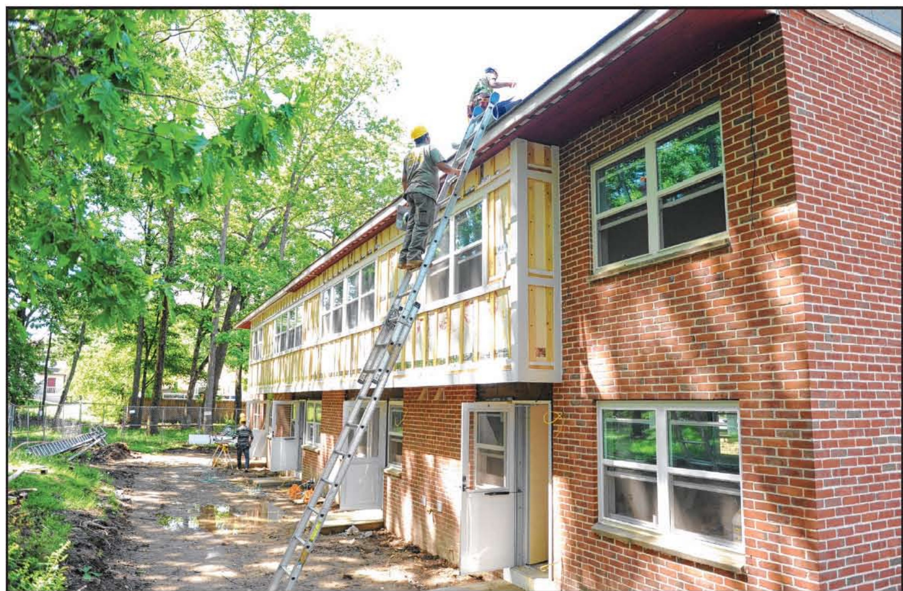
A housing unit at Oak Courts gets updated.
